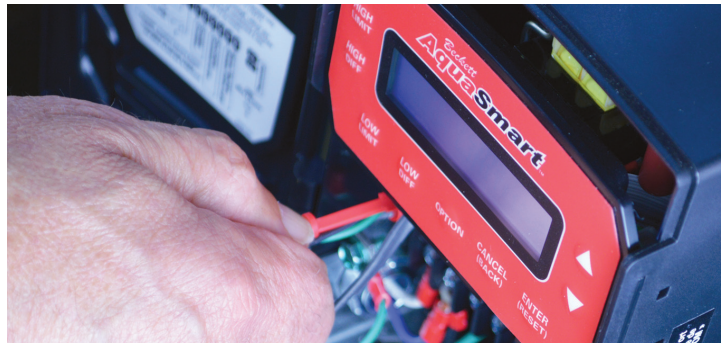
Figure 2 - Pushing Sensor into immersion well
