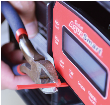
Figure 13 – Clipping the Pushrod to Length
