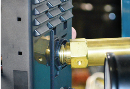
Figure 5 – Mounting to Immersion Well
