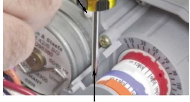
Transition Cam is set with Screwdriver
